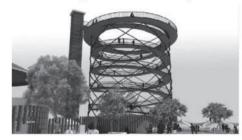
The grid-like/akin steel structural members of the Tower are, according to the firm, inspired from the bird's nest. It is further expected to give 'a sensational and dramatic effect' to the visitor as the structural members are woven and inter-woven around the ramp. One other feature of the Tower is that maximum space is provided in the deck area so that visitors could 'enjoy the grand view from the top'.
